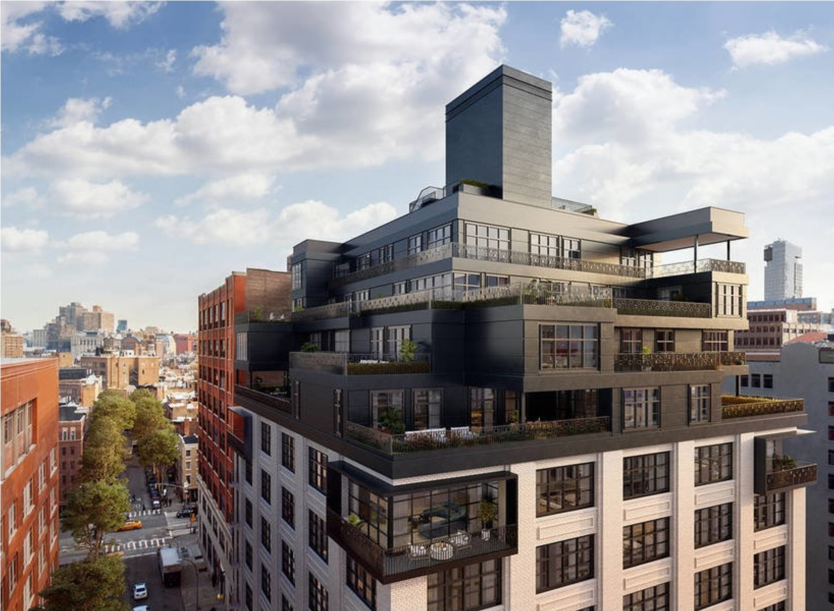
A newly constructed penthouse in 90 Morton Street in New York is asking $37.5 million. BINYAN/IF STUDIO
